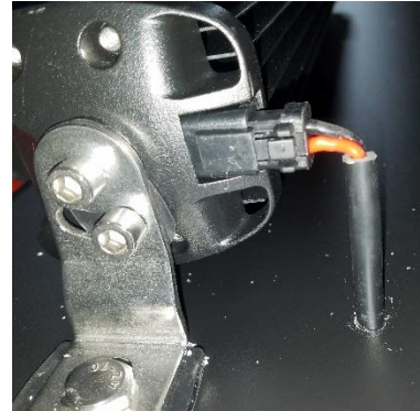
Figure 12: Routing Cable Through Roof
