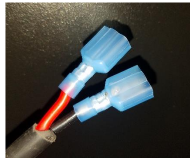
Figure 13: Spade Connectors on Light Bar Cable
