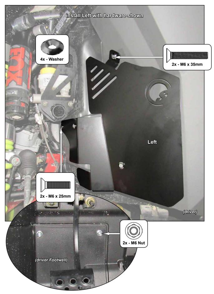
Tighten hardware completely and repeat steps for opposite side.
