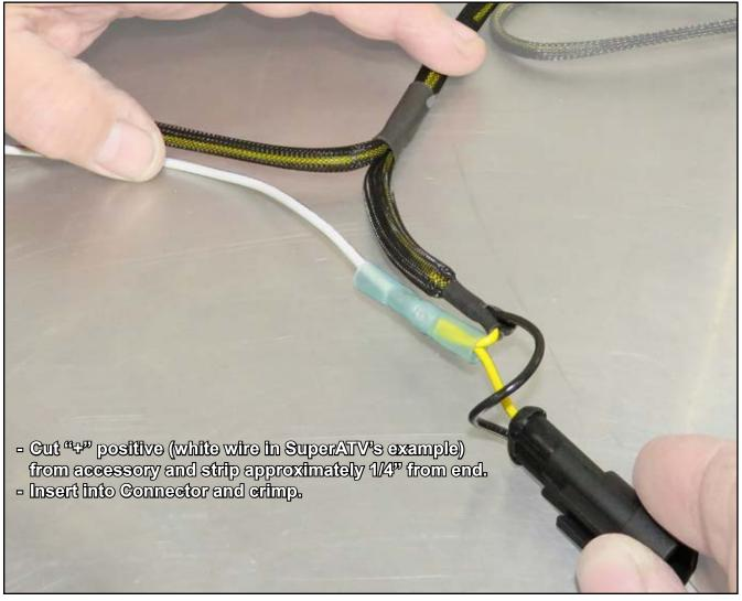
SuperATV recommends using a handheld mini torch, or lighter, to activate heat shrink on Connector.
