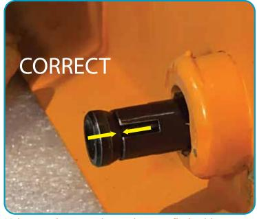
Make sure the expansion anchors are flush with no gap.
