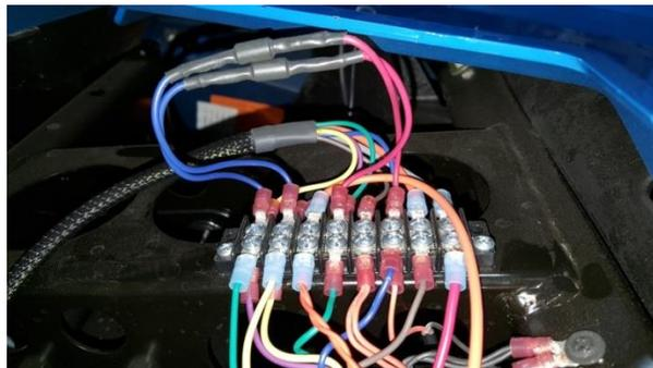
Diode jumped across circuits
